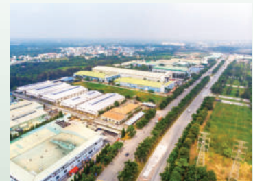
A view of Thanh Loc Industrial Zone
