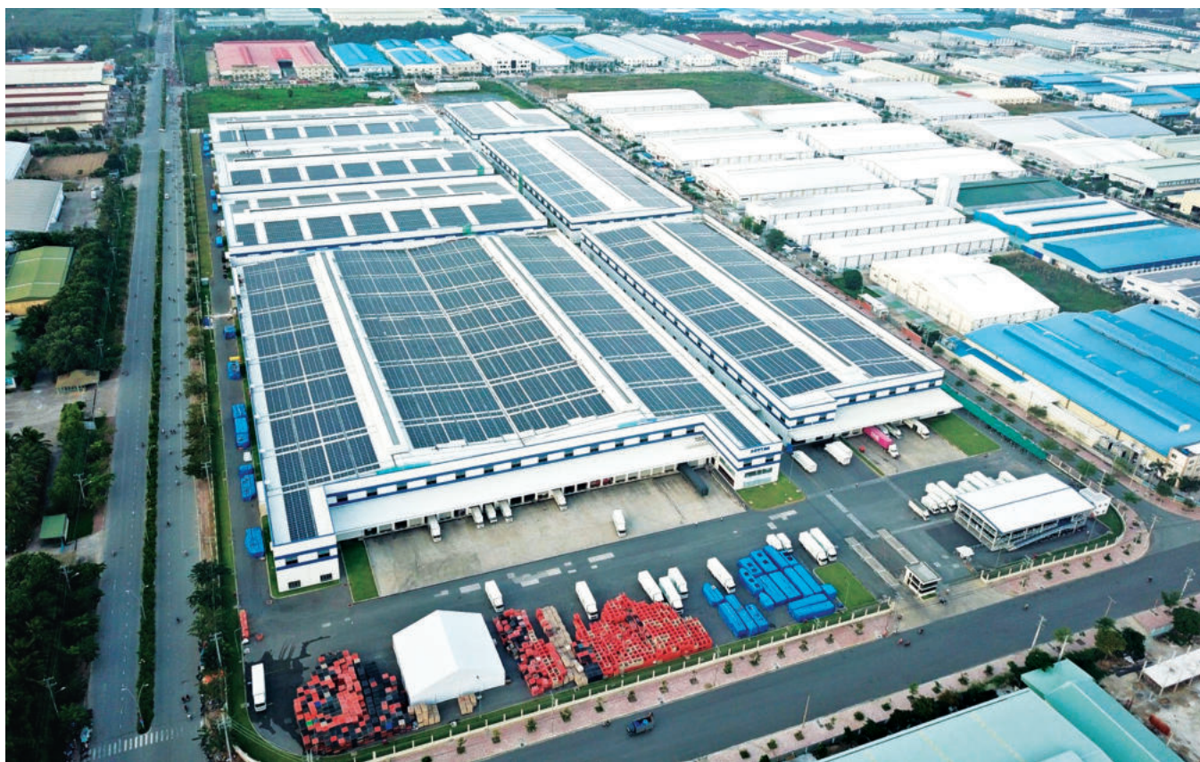
The rooftop solar power system at Duy Tan Plastics Factory is monitored and its efficiency evaluated through data collection
