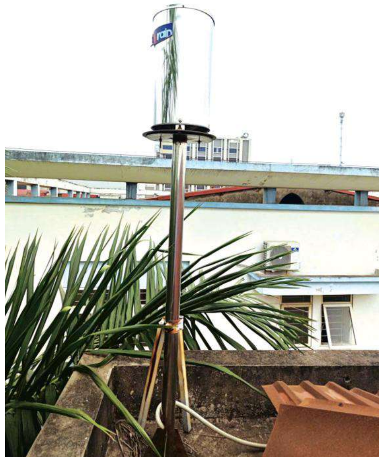
Equipment and technical cabinet of an automatic rainfall monitoring station connected to the operations center
