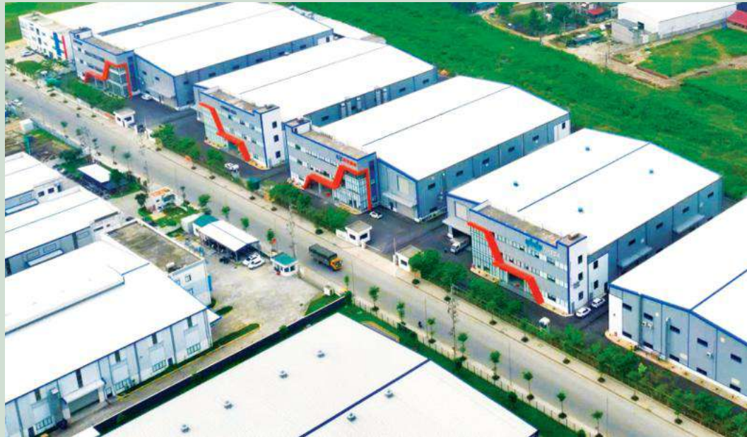
Modern factory systems in operation, demonstrating investor confidence in Thuan Thanh III Industrial Park – Sub-zone B
