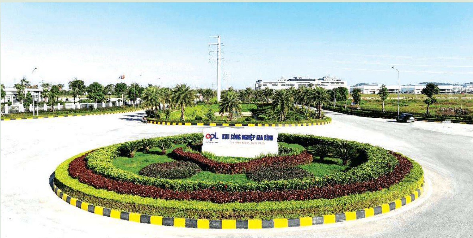
Gia Binh Industrial Park developed by Capella Land is an attractive destination for FDI thanks to its strategic location and well-developed infrastructure
