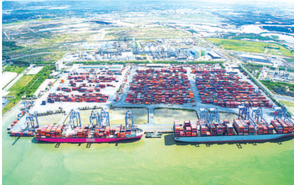
Overview of Tan Cang-Cai Mep International Terminal (TCIT)
