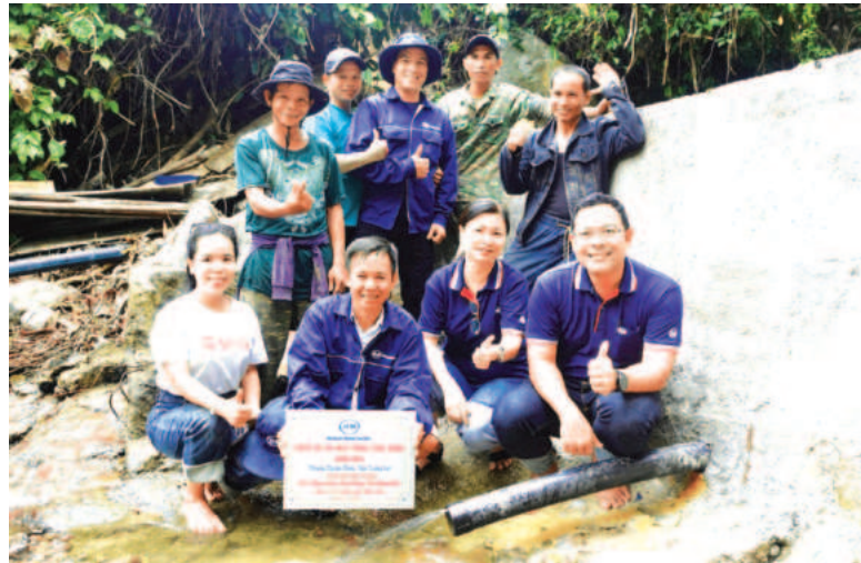
With 3,000 meters of installed water pipes, Binh Minh Plastics and SCG's Water Supply Project has improved the lives of more than 240 households in Ga Lee village
