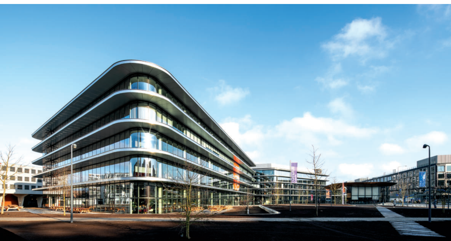
ING Cedar Building, Amsterdam
