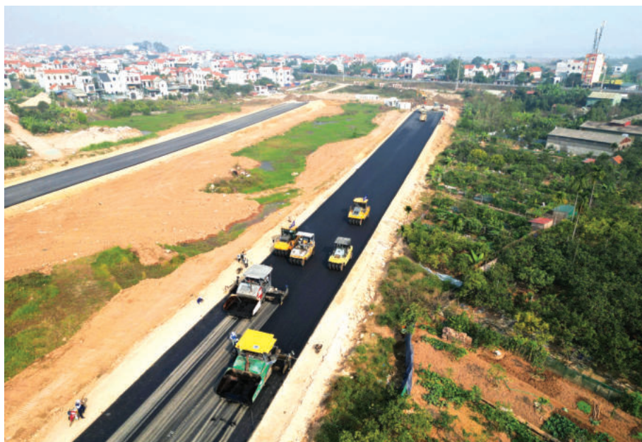
The development of socio-economic infrastructure continues to be identified as one of the three strategic breakthroughs in 2026
